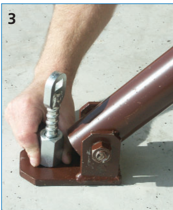
3. Tighten hexagonal bolt, in this way the nut will center the clamping part without tolerances.
