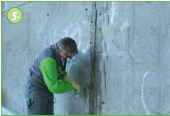
Pre-wet the crack
