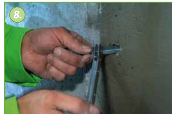
Use a wrench to tighten the packer.
