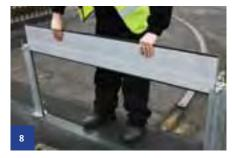
Begin inserting the first panel into the rails, ensuring that you start with the rubber sealing bottom panel first (these panels have seals on both top and bottom).
