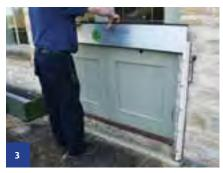
Prior to slotting in the first Aluminium Panel, please ensure that the floor surface and its immediate surroundings are free from any debris. Once this is done, you can start inserting the panels.
