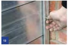
Partially tighten the horizontal compression screws either by hand or using the 6mm Allen key provided, so that panels begin to depress against the rubber seal on the inside of the channels.
