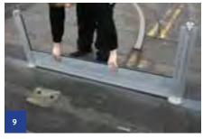
Continue the process of inserting all bottom panels along the entire barrier length.
