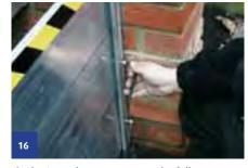
The horizontal screws can now be fully tightened followed by the tightening of top locking and end rail compression blocks using the necessary Allen key.
