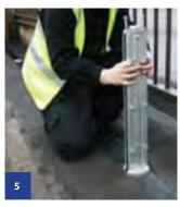
Insert demountable post into ground insert.
