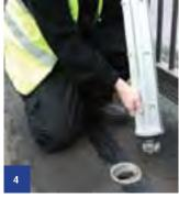
Before inserting the demountable post, please ensure that the insert and its immediate surroundings are free from any debris.
