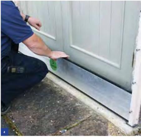
Carefully insert each panel, ensuring that you start with the rubber sealing bottom panel first (these panels have seals on both top and bottom).
