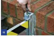
Insert fixed end rail compression blocks and partially tighten by hand or using the 8mm Allen key.
