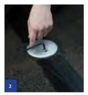
When the threat of flooding becomes apparent, commence the deployment process by unfastening ground insert dust caps with the 6mm allen key provided.
