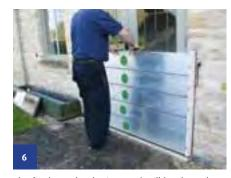
The final panel to be inserted will be the only one without rubber seals. When all panels are deployed, re-insert the Compression Blocks at the top of each Fixed Wall Rail ready for tightening.
