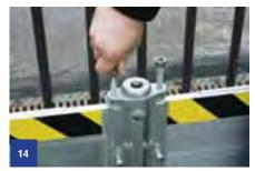
Partially tighten the vertical compression screws on the top locking block by hand or using the 8mm Allen key provided, which will depress the rubber seal on the bottom aluminium panel to the flact.
