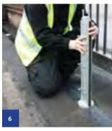
Twist demountable post 90-degrees into position to accept Panel Extrusion. Note - there is no need to tighten them in place at this stage.
