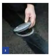
Once the caps have been loosened across the entire barrier length, lift the caps out to prepare each insert for deployment of demountable post.
