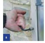
Once this is done, by using the appropriate Allen key you can now fully tighten both the horizontal screws and the compression blocks in that order.
