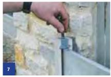
Partially tighten the horizontal screws at this stage by hand or using the 6mm Allen key provided and follow the same process for the Compression Blocks – again by hand or using the 8mm Allen key provided.
