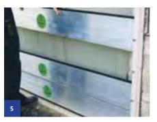
Continue the panel deployment process with the insertion of the intermediary panels (these panels have top seals on only). Note – this step is not applicable to barriers under 600mm high.
