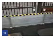
Complete the installation by inserting all other panels until you arrive at the top panel (the only panels without rubber seals).
