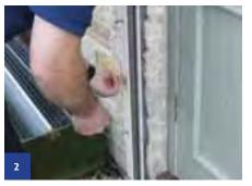
First remove the compression blocks at the top of the rails and unscrew the horizontal fixings, which are positioned down the length of the fixed wall rails. This is to ensure they do not obstruct the deployment of the panels.
